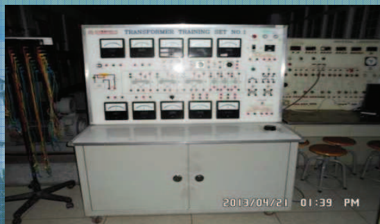
Electric Machines Laboratory
